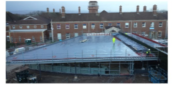
Work being done on the new Plaza at Llandough
